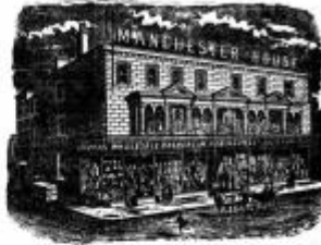
MANCHESTER HOUSE, LYNN-STREET, TODAY.
