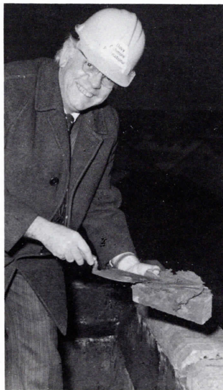
Pictured taking part in the topping out ceremony of Phase 1 at Ashmore House is Mr. T. N. Sneddon, a Davy director.
