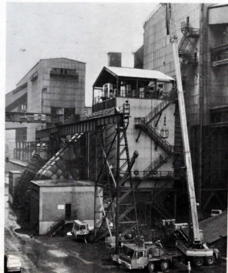
BSC Scunthorpe Appleby Frodingham Sinter Plant main strand precipitator nearing completion.
