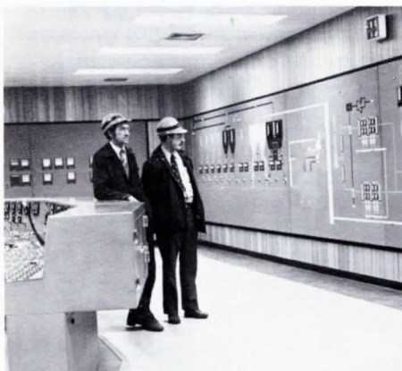
Ellis Page and Fred Ely of HWPEL in the control room at Ravenscraig.
