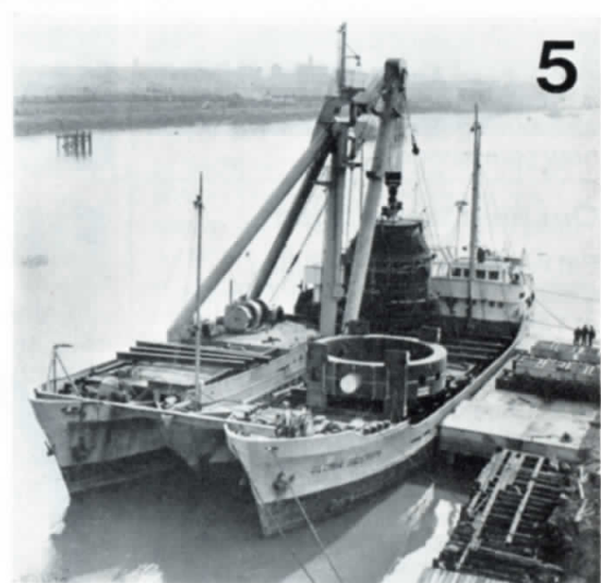
5 the Head Wrightson quay: the first shell and ring were taken round the coast 'south about' by the Gloria Siderum in April (a 680 mile journey which took three days) and unloaded three miles from Llanwern onto ...
