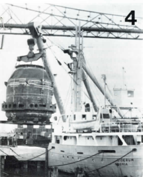
4 loading onto the ship: a specially constructed heavy lift ship with three hulls which collected the trunnion ring first from Middlesbrough Docks and then picked up the converter shell at ...
