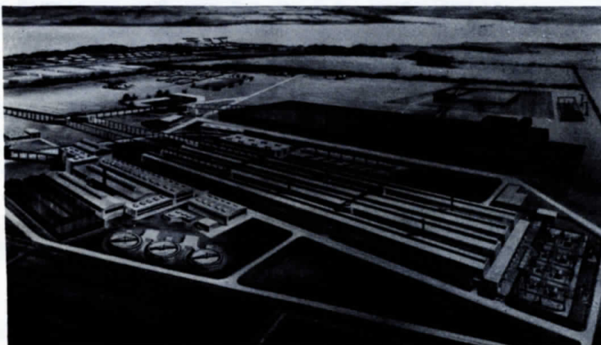
Illustration of the layout of the proposed British Aluminium Smelter at Invergordon. The "ghost" buildings indicate areas of planned expansion. This view is from the north looking towards the town of Invergordon and across the Cromarty Firth to the Black Isle.
