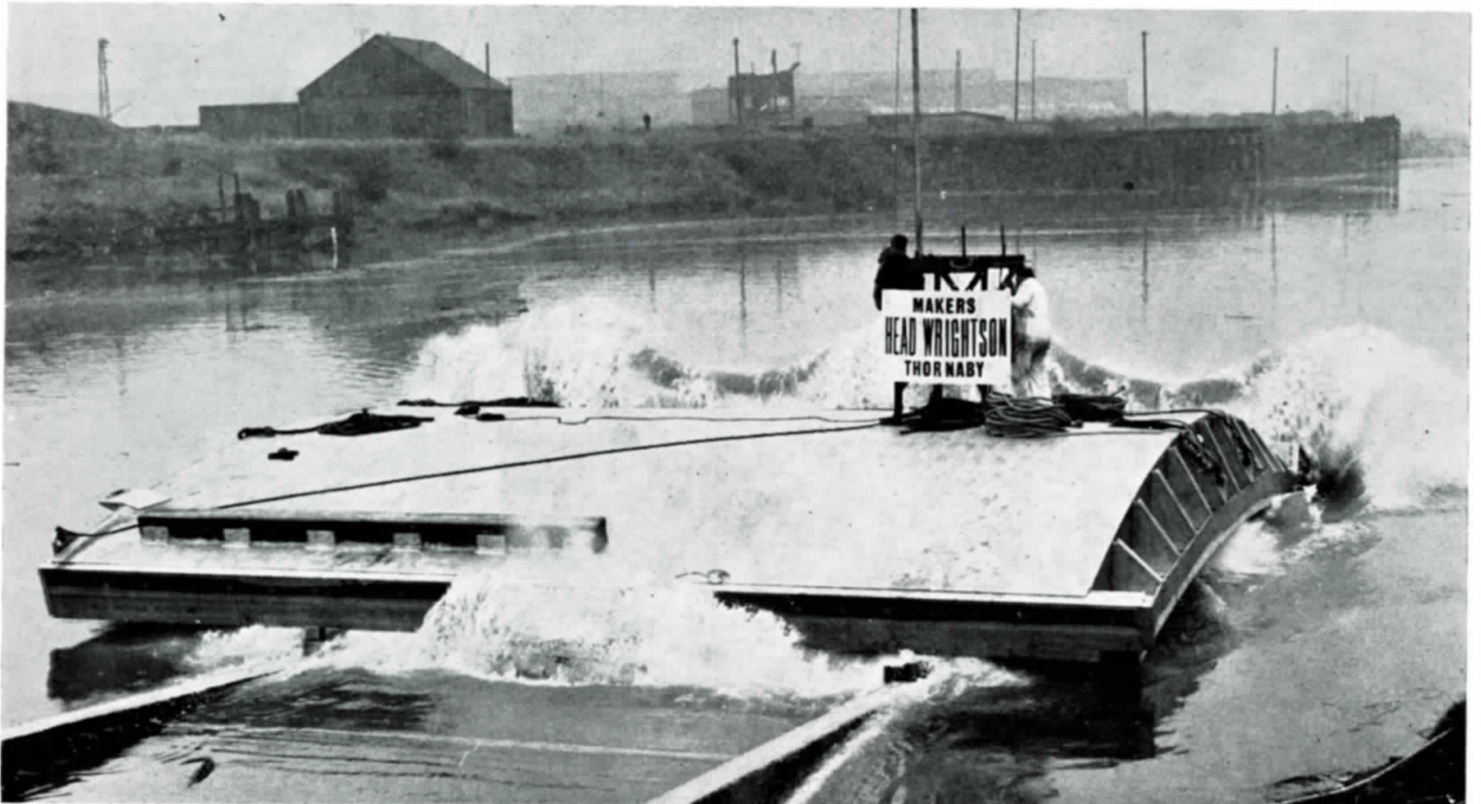
One of a pair of dock gates for the Herculeum Dock of Mersey Dock and Harbour Board being launched into the River Tees at Teesdale Works.
