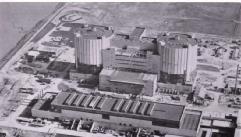
The aerial photograph opposite is of the Oldbury Nuclear Power Station which went into production early in November. For this station Head Wrightson supplied a very substantial part of the equipment.
