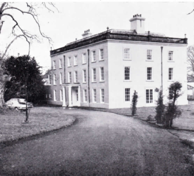
Front and side view of The Friarage.
