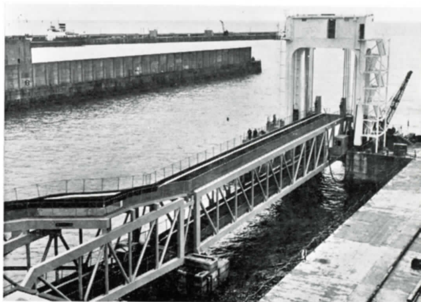
Twin level car ferry ramp at Dover
