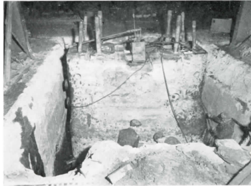
Jacking up cast steel anvil block
