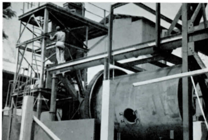
The ball mill at Carasco under construction
