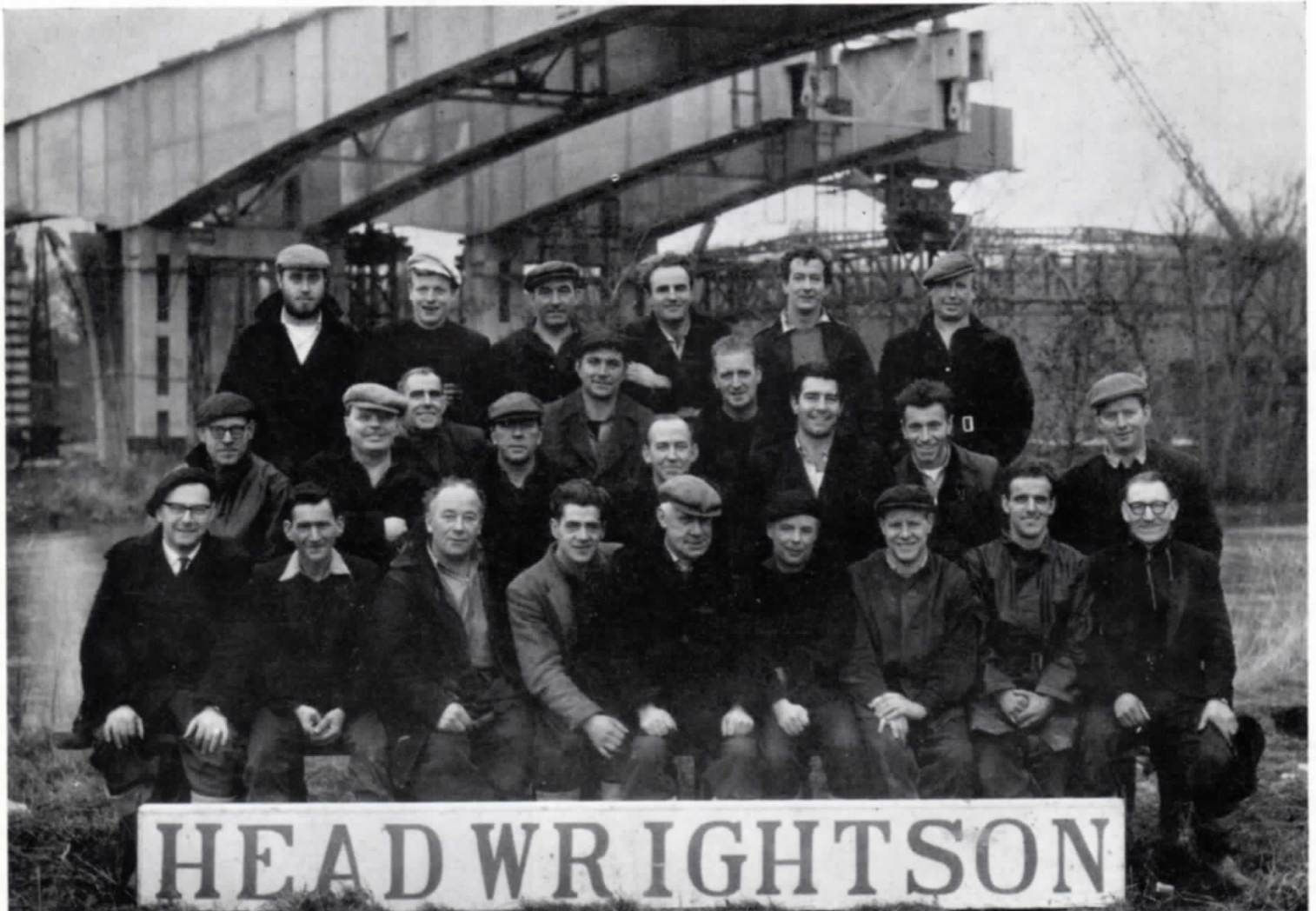
Bill Chapman and his cheerful gang of erectors after the completion of two spans of the Rossspur Bridge
