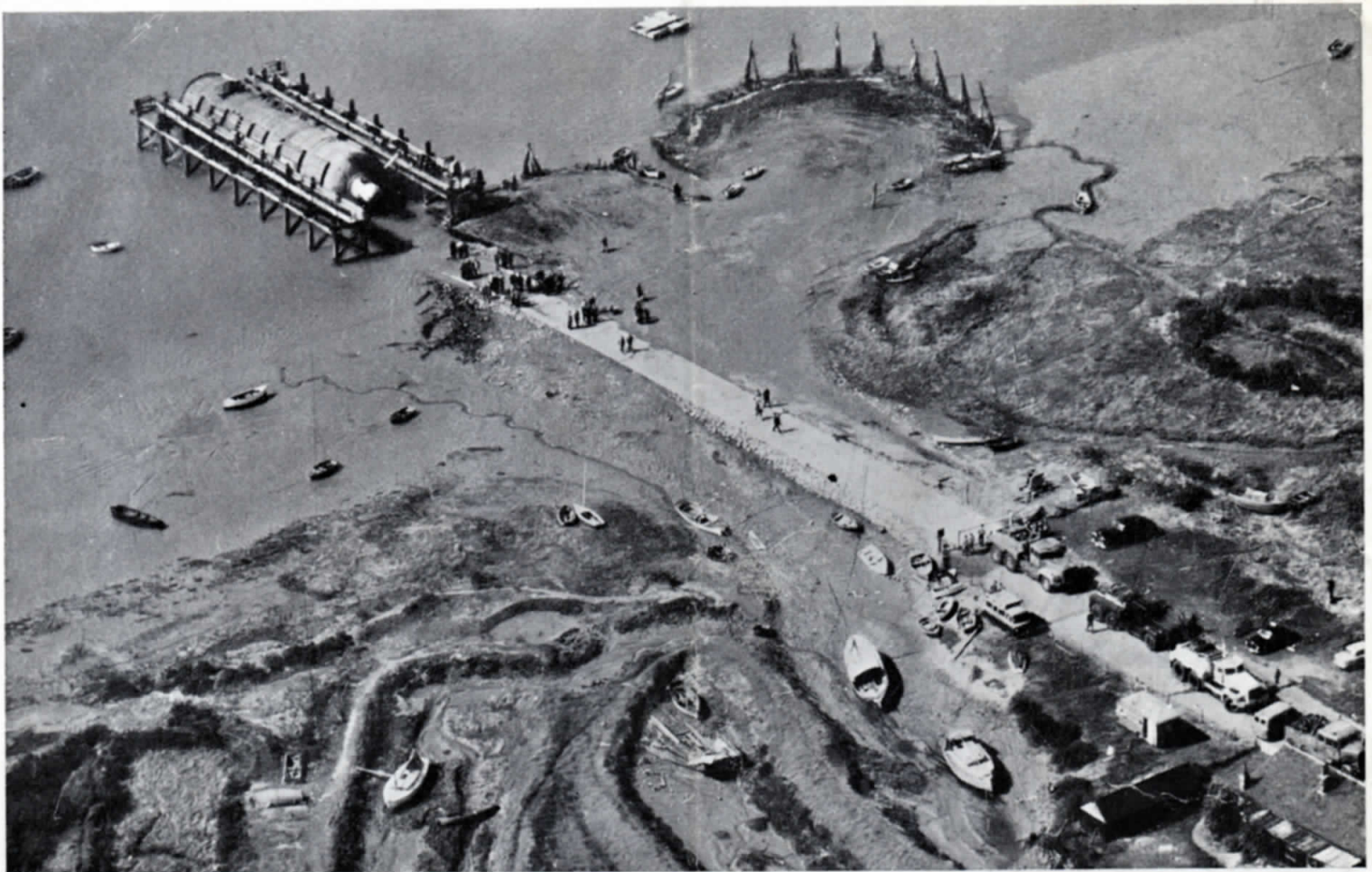
Heat Exchanger Shell on arrival at Bradwell, taken from the air
