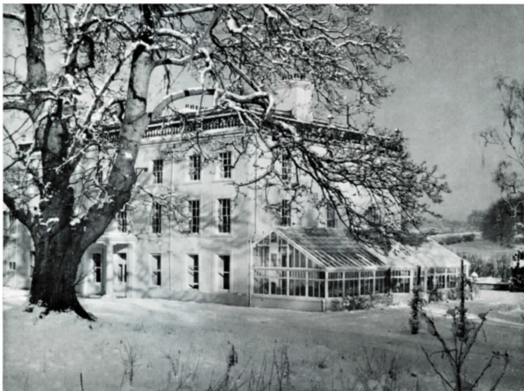
Winter view of the offices of Head Wrightson's NUCLEAR POWER DIVISION, The Friarage, Yarm, Yorks.
