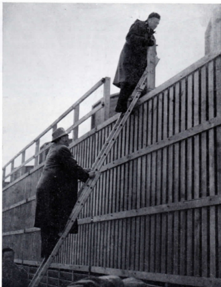
Russian Minister inspecting Cooling Tower at Harwell
