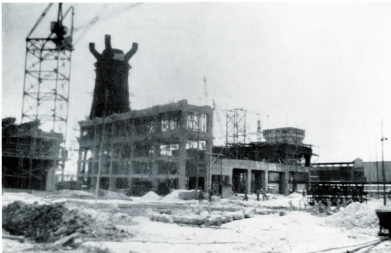
Blast Furnace Plant at Aviles
