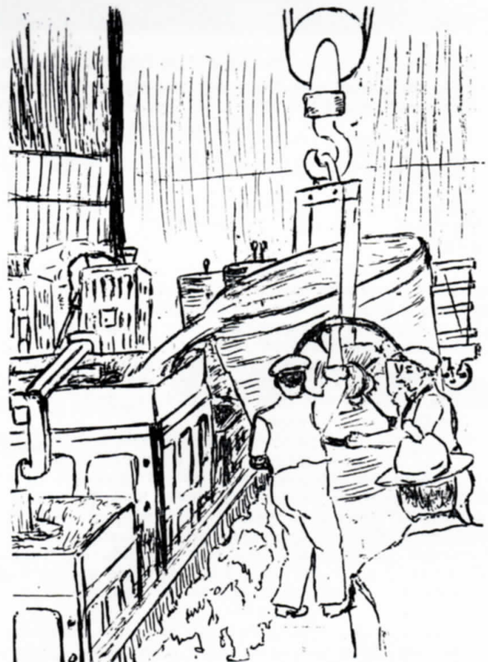
Casting a 17 ton ingot mould
